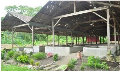
Vermi-composting facility. This provides natural fertilizer for the entire farm. It produces about 12,000 pesos/month of fertilizer.
